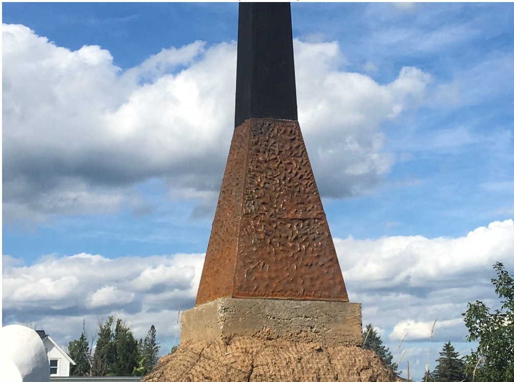
Finished Casting Weighing 150lbs, wooden spire added separately
